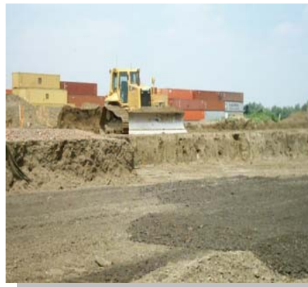
100 ha logistics park under development
