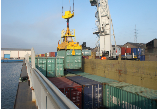
Manuport Container Terminal - Antwerp
