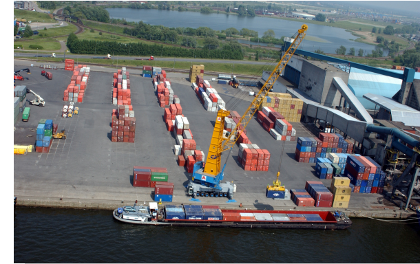
Manuport Container Terminal - Antwerp
